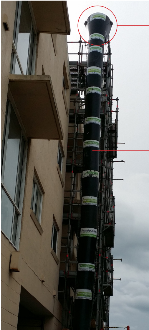
Mounted on Scaffold
